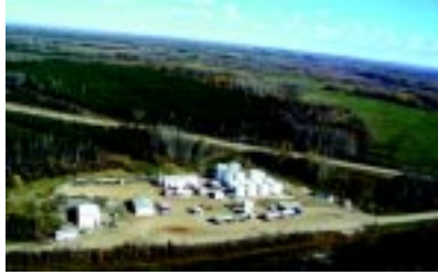
Aerial View of Plant 6
